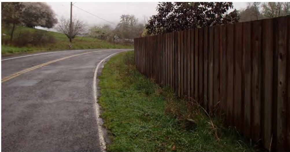
Figure 3. Area of minimum sight distance (184') heading south occurred from this point in the curve.
