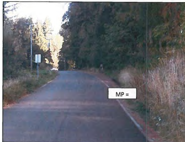
Figure 5. Roadway after the MP = 2.95, close to the end of the road (MP = 3.044).
