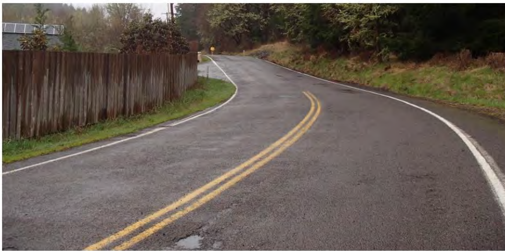
Figure 2. Area of minimum sight distance (210') heading north occurred from this point in the curve to just north of the peak of the hill.
