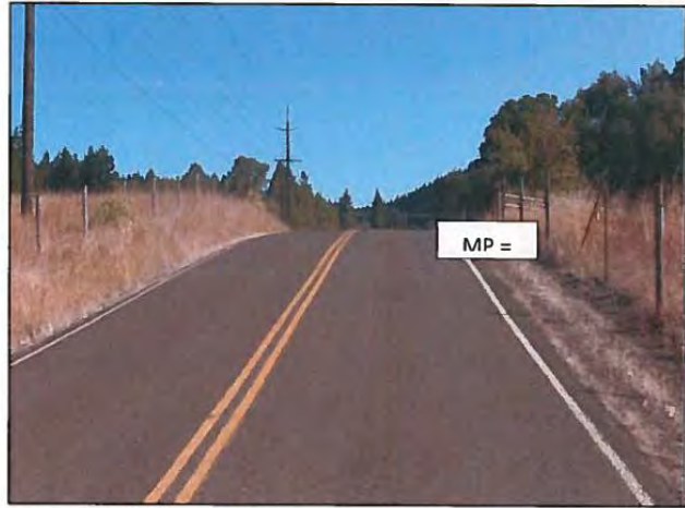
Figure 4. Visibility limitations due to vertical curve approach (MP=2.15).
