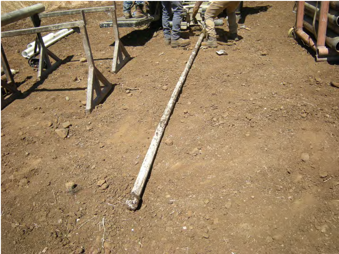
Photo A-4 – Five-foot long screen and blank casing of original well.
