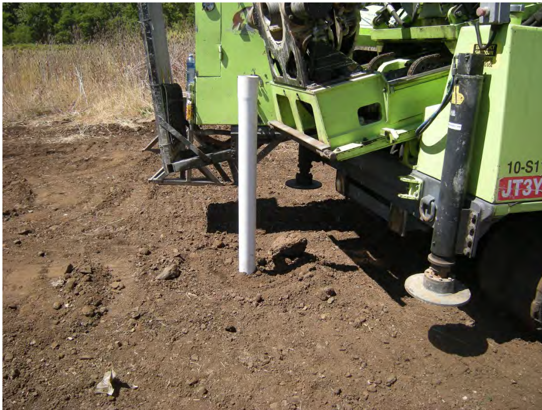
Photo A-2 – 4-inch diameter PVC protective casing in fill.
