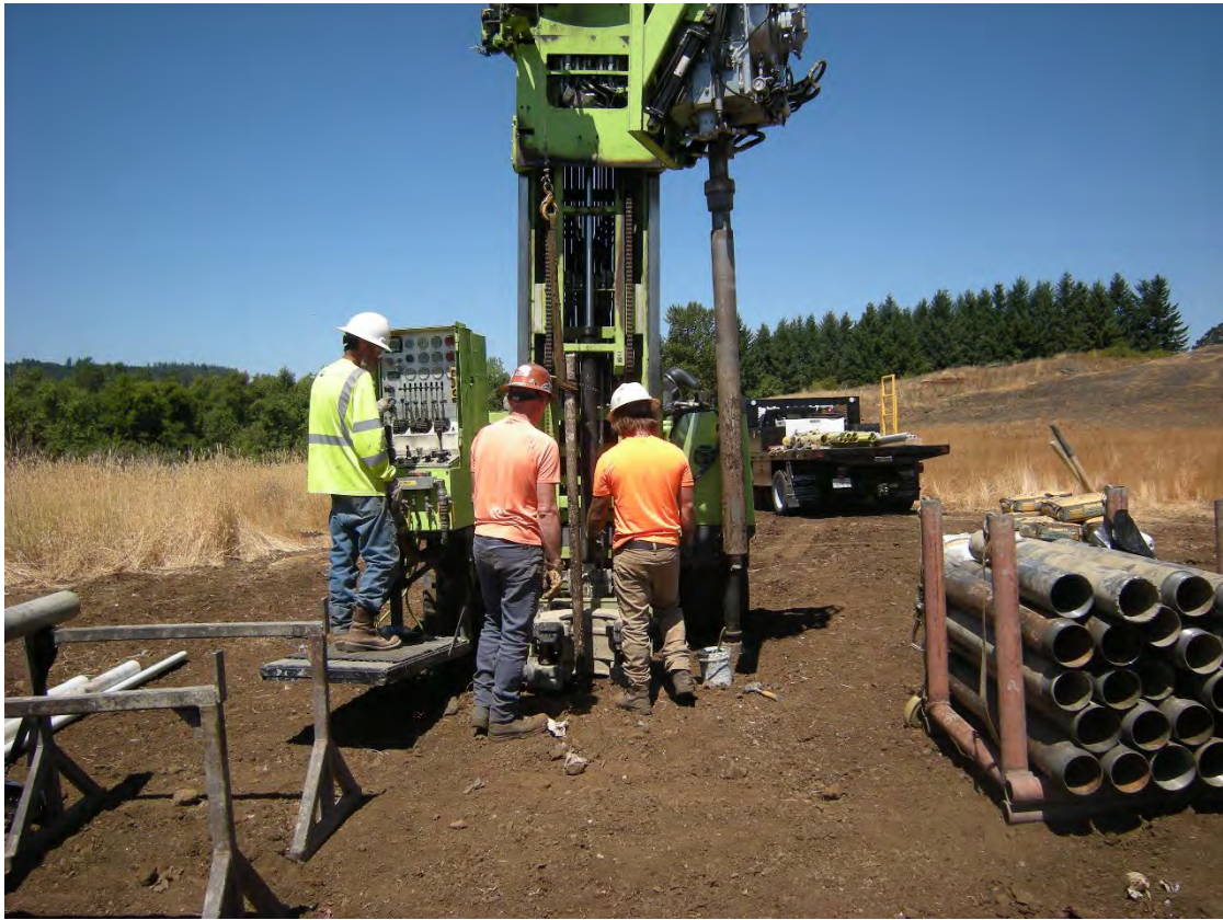
Photo A-3 – Drillers pulling original casing and screen with winch.
