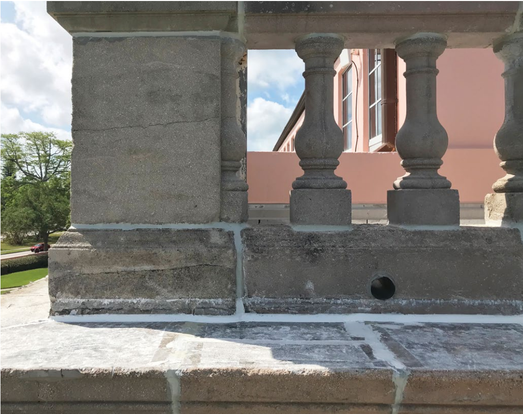
Figure 17. The balustrade consists of multiple prior campaigns of using cast stone to replace the natural stone. The effective match for the surface texture and color of the original stone allowed individual elements to be incrementally replaced only when they had failed, thus retaining the maximum amount of original material as long as possible. Photo: EverGreene Architectural Arts.
