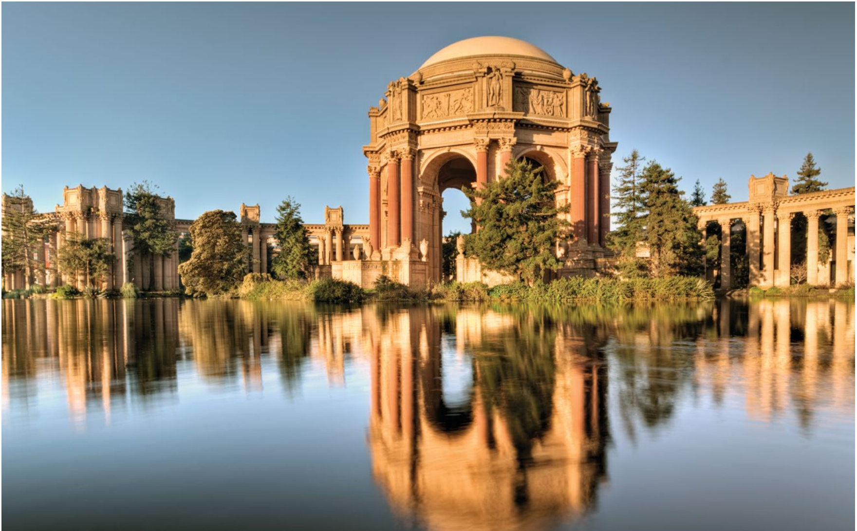
[8] The Palace of Fine Arts was designed by Bernard Maybeck and built for the 1915 Panama-Pacific Exposition in San Francisco. The pavilion was intended to be temporary and, although it had a steel structure, the exterior was finished only with stucco, an impermanent material composed of plaster and fiber. The building was not torn down after the exposition, and it eventually fell into ruin. In 1964, all but the steel structure was demolished, and the building was reconstructed with lightweight poured-in-place concrete. Photo: KevinIcole at Wikimedia Commons.
