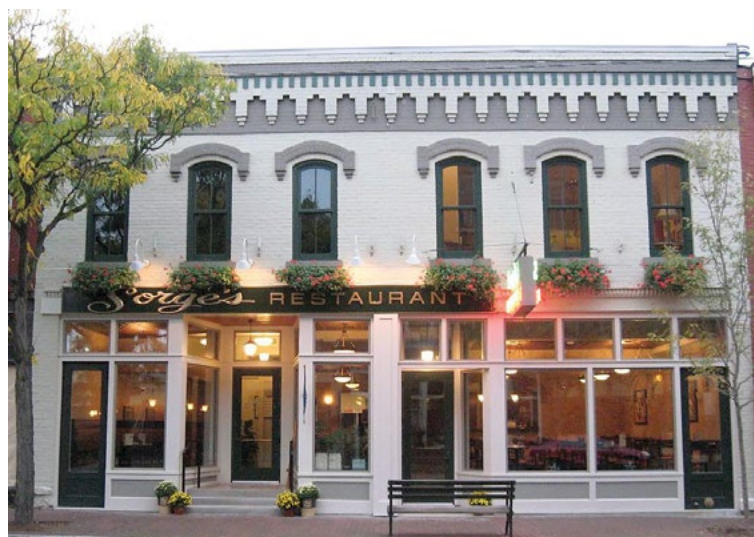
[28] This new storefront, which replaced one that was missing, is compatible with the historic character of the building.
