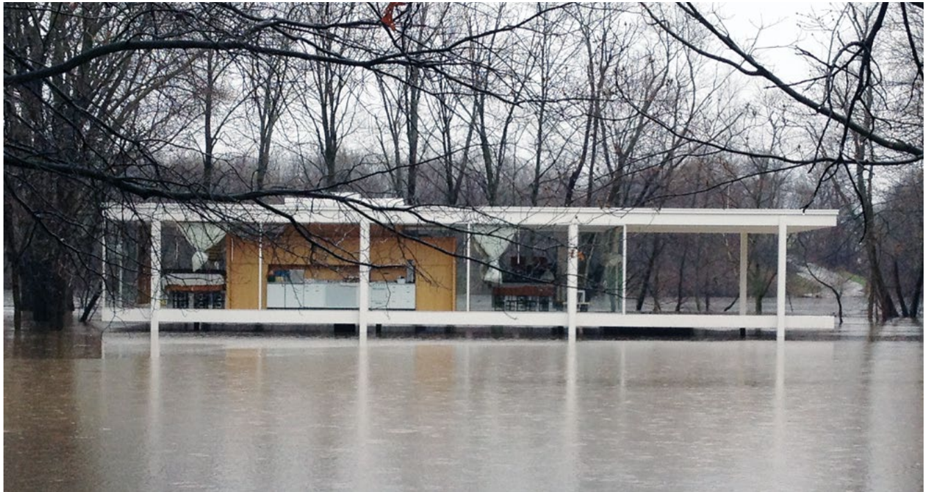
[19] The 1951 Mies van der Rohe-designed Farnsworth House, Plano, IL, was built close to the Fox River, which is increasingly prone to floods. To preserve the house in its original location, historic preservation architects and engineers continue to explore ways to protect it from the flooding, including a possible system that would lift the house above the flood waters and lower it back to the ground. Photo: Courtesy Farnsworth, A Site of the National Trust for Historic Preservation.
