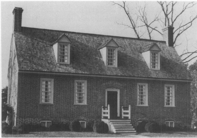
1. The Rolfe-Warren House, a tidewater Virginia property, was restored to its 18th-century appearance in 1933. The handsplit and dressed wooden shingles are typical of the tidewater area with special features such as curved butts, projecting ridge comb and closed swept valleys at the dormer roof connections. Circa 1970 Photo: Association for the Preservation of Virginia Antiquities.
