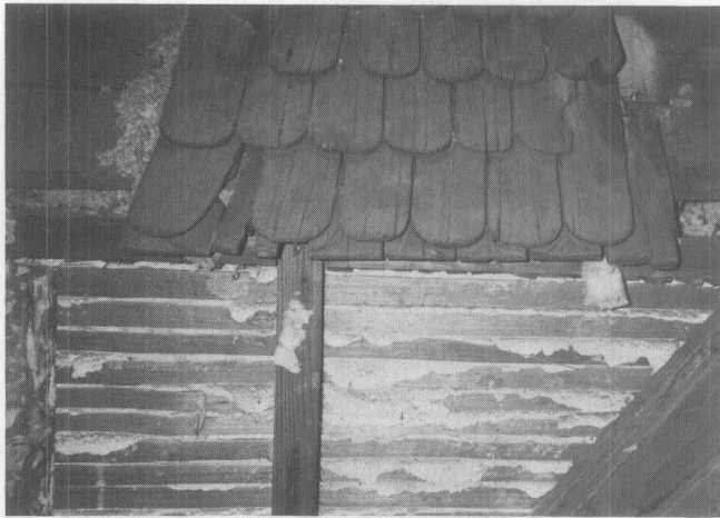
B. These weathered historic 19th-century handsplit and dressed shingles were found in place under a later altered roof. Note the straight butt eave shingles under the curved butts of the historic dormer shingles.
