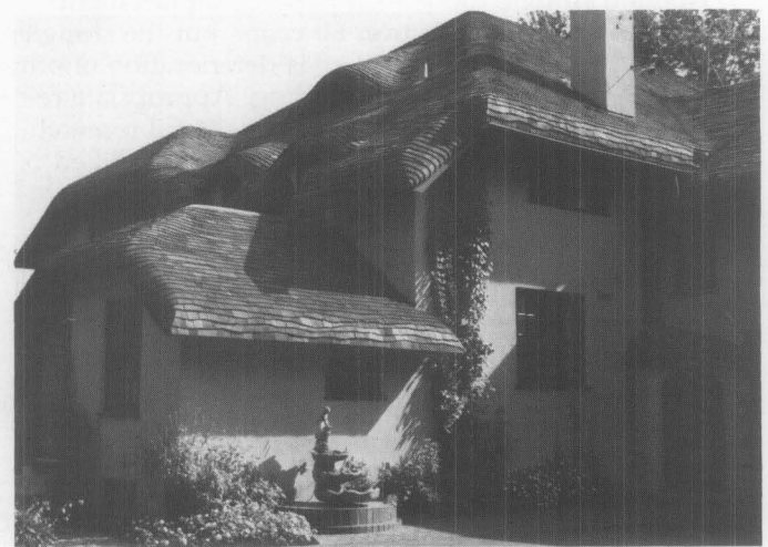
4. With the popularity of the revival of historic styles in the late 19th and early 20th centuries, a new technique was developed to imitate English thatch roofs. For the Tudor Revival thatch cottages, steaming and curving of sawn shingles provided an undulating pattern to this picturesque roof shape. Photo: Courtesy of C.H. Roofing.
