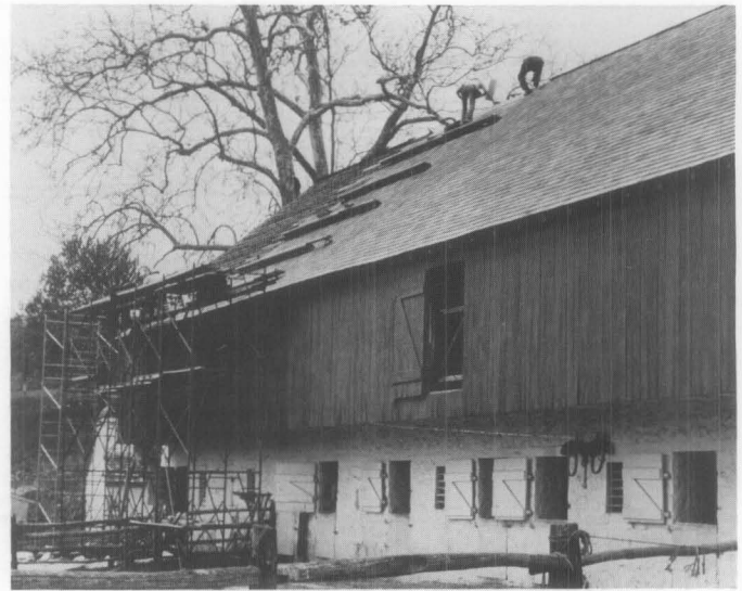
11. The replacement sawn red cedar shingles matched the deteriorated shingles exactly for this barn re-roofing. The old shingles, seen to the far left, were removed as the new shingles were installed. Even the horizontal coursing matched because the exposure length for both old and new shingles was the same. Photo: Williamsport Preservation Training Center.
