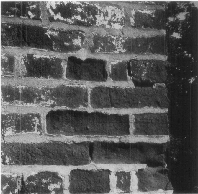
Figure 5. The use of hard, portland-cement mortar that is less permeable than the soft bricks has resulted in severe damage to this brick wall. Moisture trapped in the wall was unable to evaporate through the mortar which is intended to be sacrificial, and thus protect the bricks. As a result the moisture remained in the walls until water pressure eventually popped the surface off the bricks. Photo: National Park Service Files.
