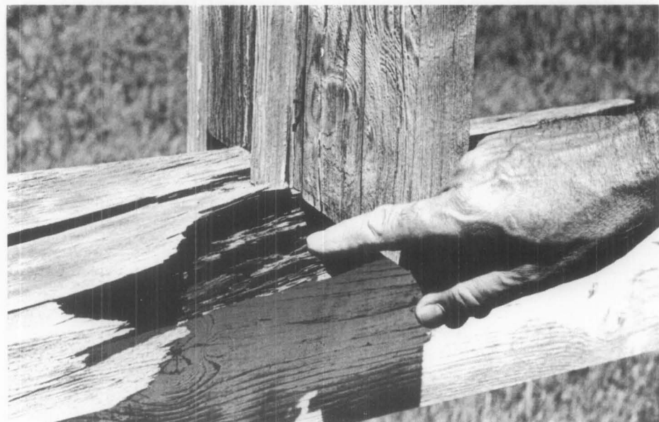
Figure 2. Close-up view of decayed, untreated window frame. Frame fell apart after 6 years' exposure. Photo: Courtesy of the Forest Products Laboratory
