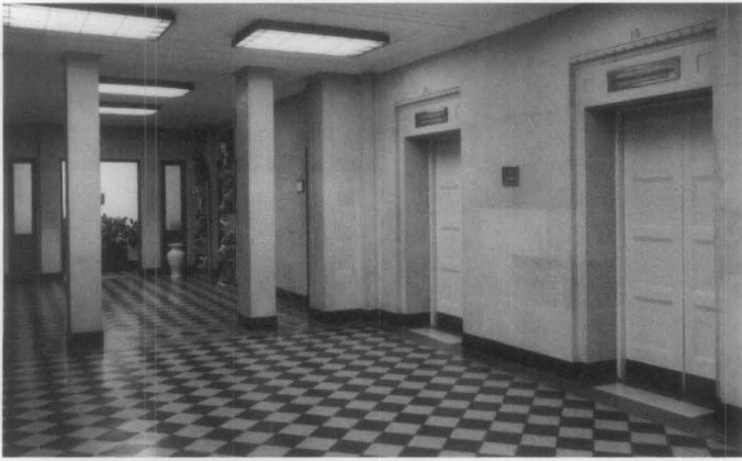
Figure 13. Quarry tiles were used in the corridors on many of the upper floors of the U.S. Department of the Interior Building (1935-1936). They were laid in a pattern identical to the more expensive marble floor tiles that were used in the public spaces. Photo: Brooks Photographers, HABS Collection.
