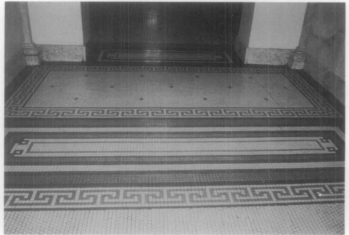
Figure 11. Ceramic mosaic tiles were used decoratively on the entrance floor of this early-20th century school building. Photo: Kimberly A. Konrad.
