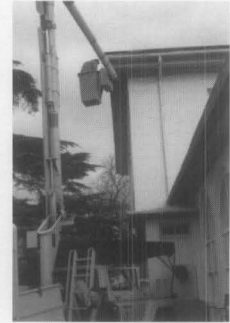
A. Inspecting the overall building on at least an annual basis will identify areas needing maintenance. A bucket lift is helpful for large buildings. Photo: author.
