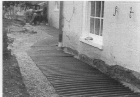
A. Mitigate poor drainage with gravel, filter cloth, or the use of subsurface drainage mats under finished paving. Photo: Larry D. Dermody.
