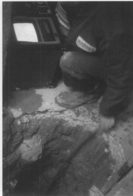
Fig. 16. Contractors specializing in building diagnostics often have video camera or fiber optic equipment that allow the viewing of inaccessible areas. This is particularly helpful in chimney flues or subsurface drains, as shown here. In the past, these areas would need to be excavated for visual inspection. Photo: author.
