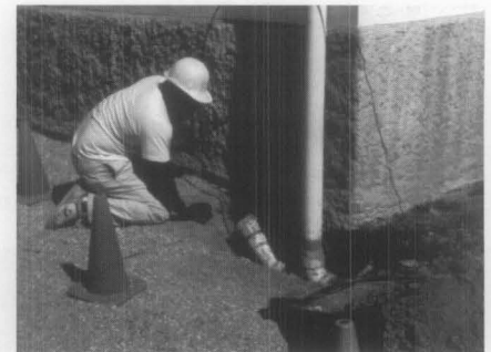
C. Cleaning out gutters and downspouts should be done at least twice a year. Photo: WPTC, NPS.
