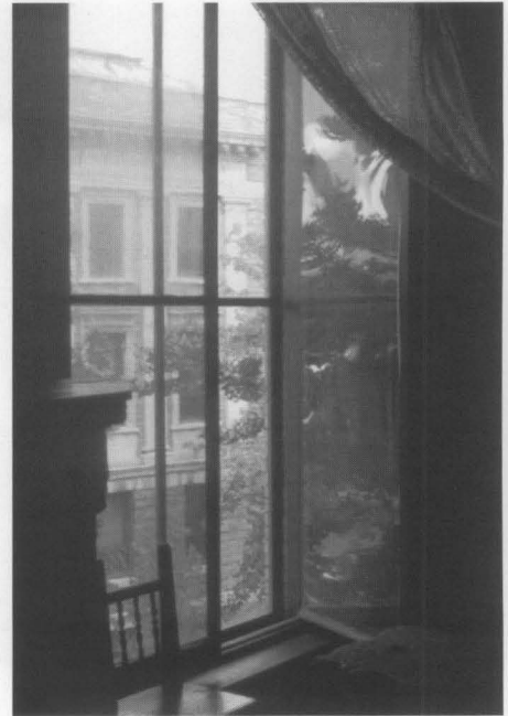
F. Triple glazed windows replaced the originals to control condensation. Photo: © Isabella Stewart Gardner Museum, Boston.
