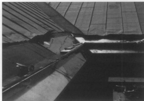
B. Repair roofs and add ice and water shields at eaves and under valleys in cold climates. Photo: Larry D. Dermody.
