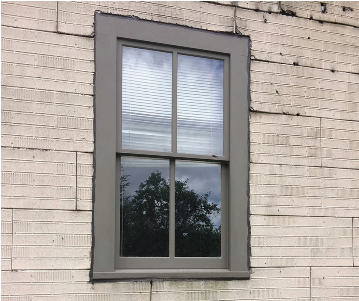
Asphalt/fiberboard siding, trade named Insulbrick, applied in the 1940s to an 1880s miner's cottage.
