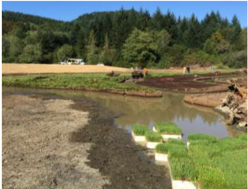
Figure 3-9 Installation of wetland sod
