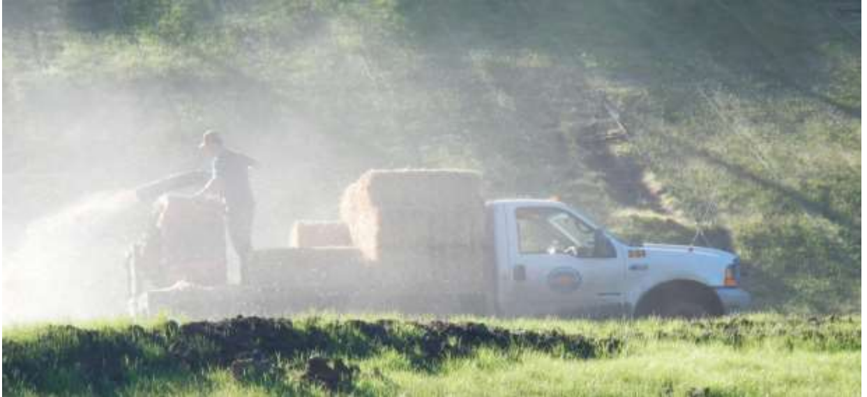
Figure 3-5 Straw Mulch being blown on site
