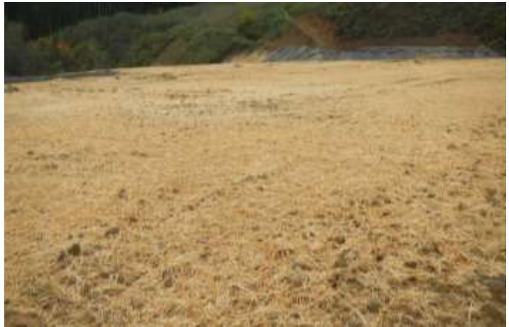
Figure 3-6 Good cover with straw mulch
