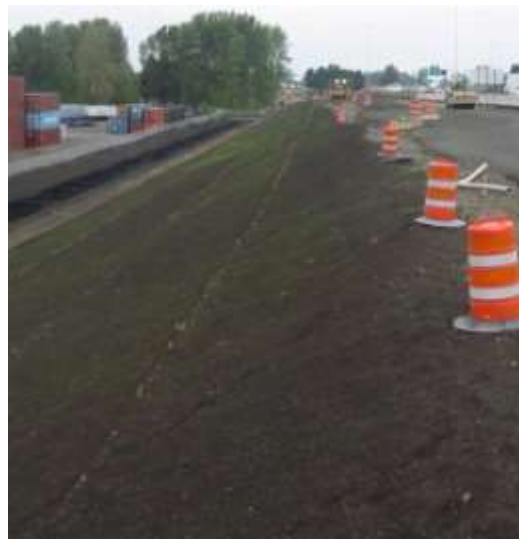
Figure 2-9 Compost blankets provides erosion prevention
