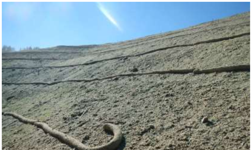
Figure 3-22 Fiber Rolls (Wattles) – Sediment Barrier Type 3
