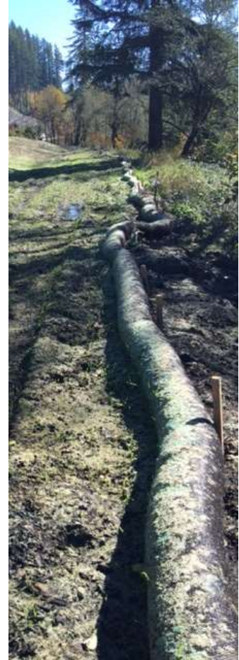
Figure 3-23 Compost Sock – Sediment Barrier Type 8
