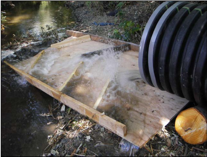
Photo example of Wood Sheet Energy Dissipator
