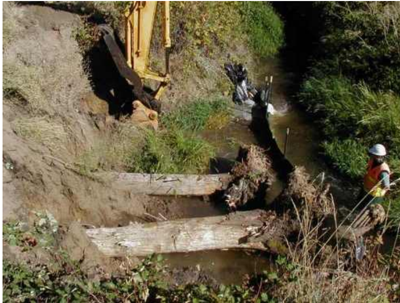
Photo example of Working in the Wet
