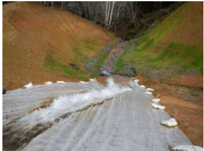
Figure 3-15 Plastic sheeting used as Temporary Slope Drains
