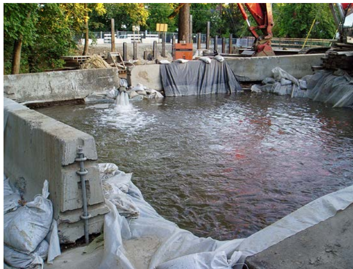
Photo example of Sediment Trap
