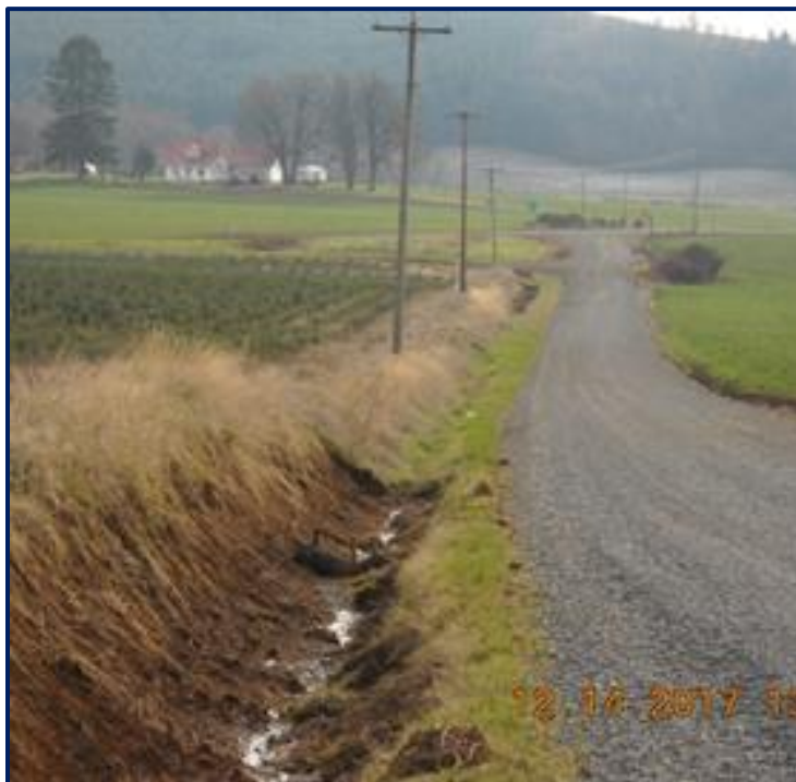
Skip ditching in action along a rural roadway.
