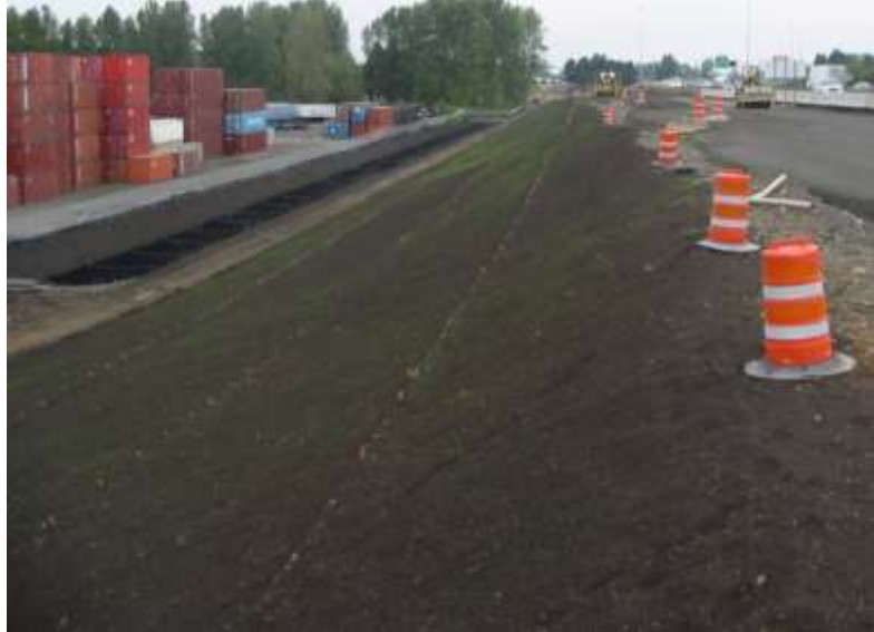
Figure 3-12 Compost blankets provides erosion prevention
