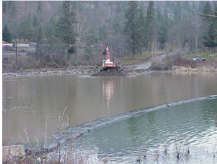
Photo example of Silt Curtain
