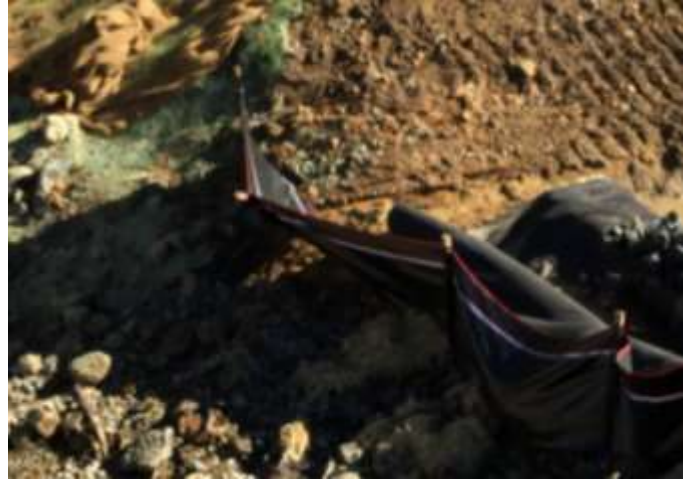
Figure 3-30 Sediment fence not embedded in ground
