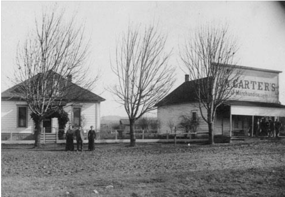
Downtown Wellsdale in 1941, shortly before the town was demolished to make way for Camp Adair. Photo by Ben Maxwell (part of the Ben Maxwell Collection, Salem Library).
