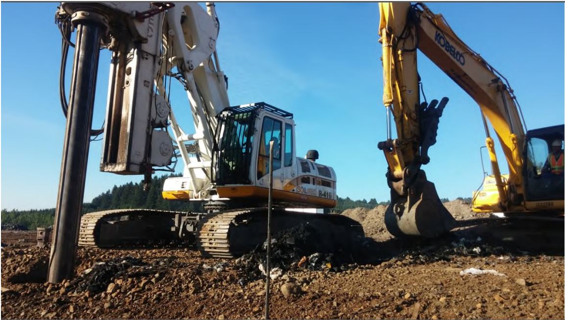
Figure 2. Vertical Gas Well Construction
